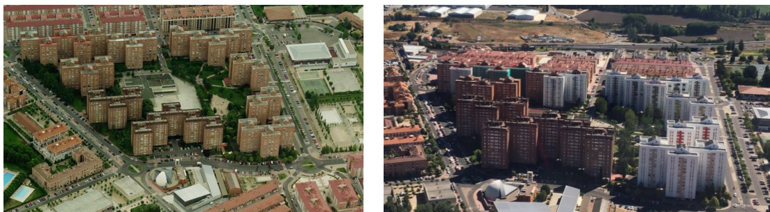
Figure 5. Torrelago district: Original buildings (left) and retrofitting process (right)
