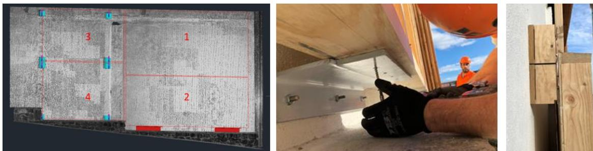
Fig. 3. Left: Identification of the zones for the distribution of the modules in the wall; Center: Strategy 1: traditional installation system; Right: Strategy 2: installation with the Matching Kit system [Source: BERTIM project]
