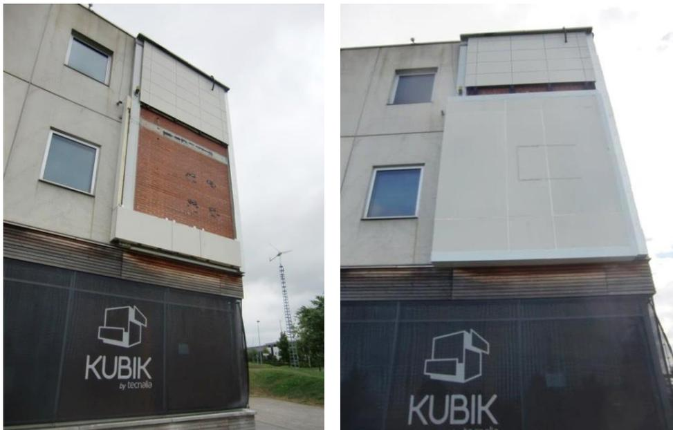
Fig. 1. Test area at first floor of west-facing façade in KUBIK facility: (a) original brick wall before installation; (b) ETIXc prototype installed.
