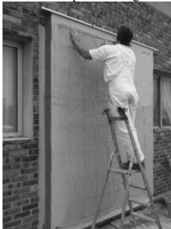
Fig. 3 Capillary tubes within a render finish [2]
